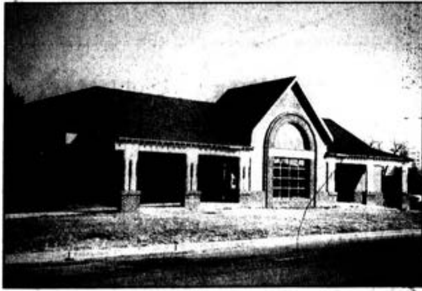
This new addition to Three Lower Counties Community Services in Princess Anne recently opened.
