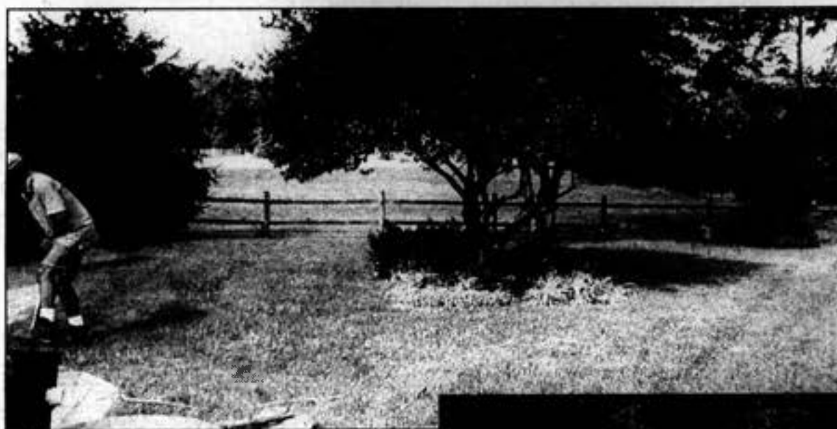
This backyard site was transformed into a decorative pond in just 12 hours. Ground was broken at 8:30 a.m., above. After the digging was completed, the liner and stones were put in place, right. By 8:30 p.m. that same day, the pond was finished, complete with plantings and mulch.
