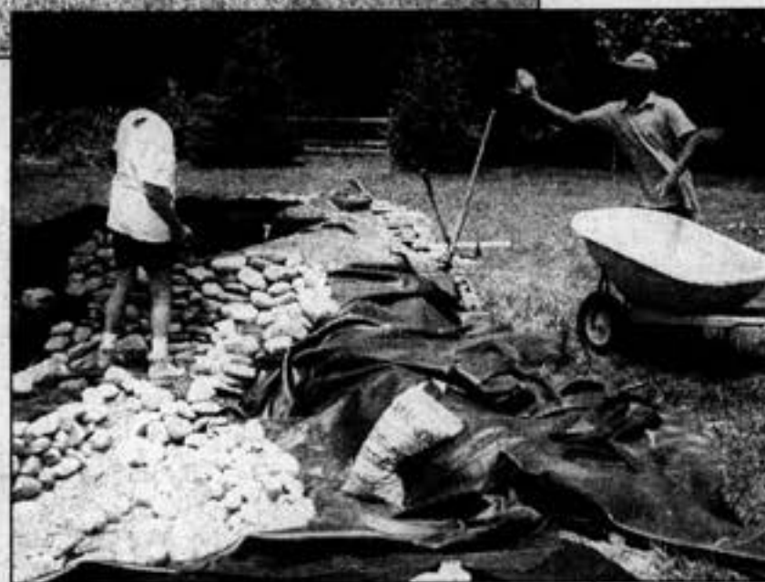
This backyard site was transformed into a decorative pond in just 12 hours. Ground was broken at 8:30 a.m., above. After the digging was completed, the liner and stones were put in place, right. By 8:30 p.m. that same day, the pond was finished, complete with plantings and mulch.
