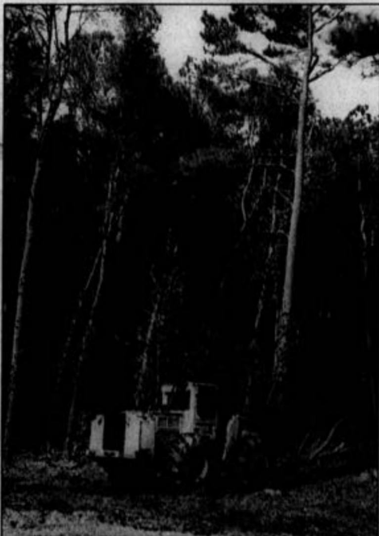
Land is cleared for a new development on Dryden Road in Princess Anne.
